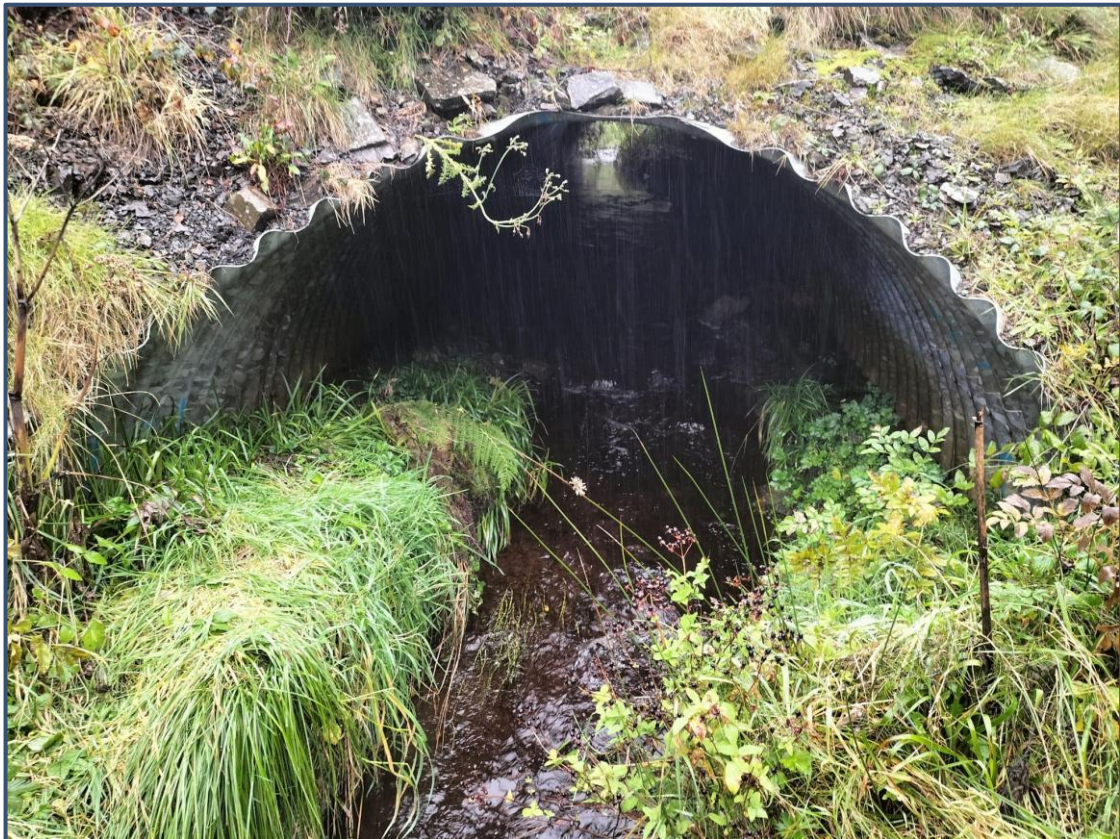
Plate 4-38. The culvert at survey location GC3.
